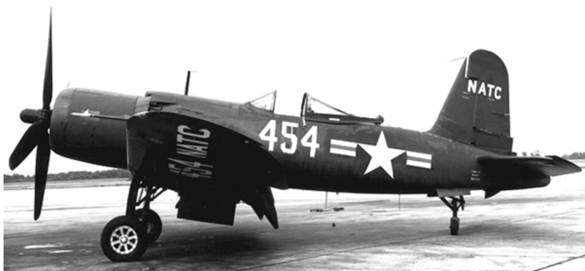
With its massive 3,000 hp. engine, the F2G Corsair was pure muscle. It reportedly could climb to 30,000 feet in less than five minutes. (Courtesy Bob Lawson)
